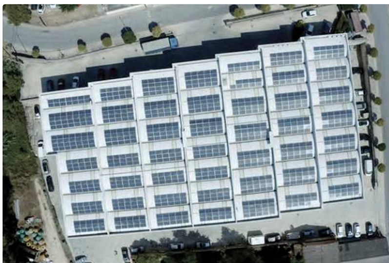
Energy self-supply from solar panels. Autoconsumo di energia attraverso pannelli solari.
